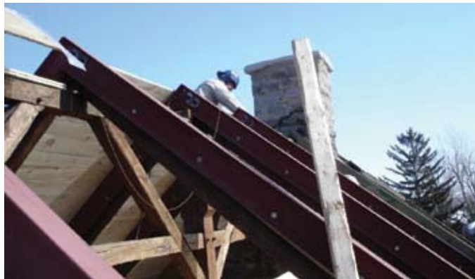
Reinforcing historic heavy timber roof structure with steel members.
