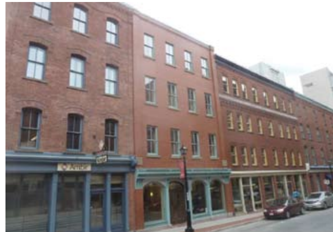
New Construction (infill) fills former void in streetscape and is designed sensitively in context using compatibly-sized windows and materials. Source: Jim Bezanon
