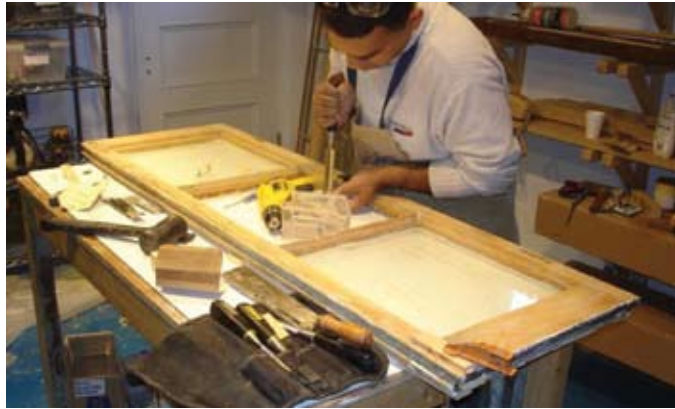
Rehabilitating a wood window. Source: FGMDA
