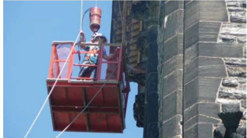
Figure 79 Inspecting masonry. Parliament Hill. Ottawa, ON. Source: MTBA Associates Inc.
