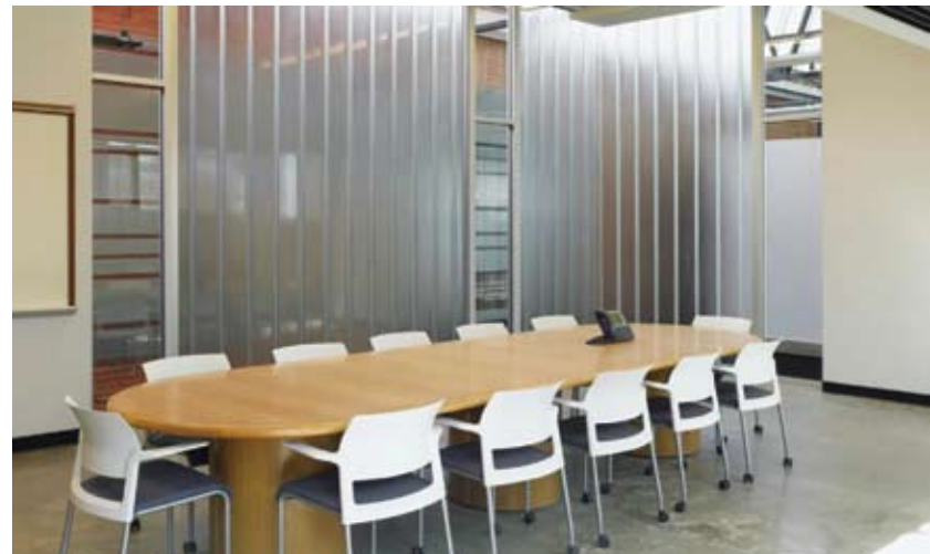
Figure 74 New glazed partitions used to enclose meeting room, allowing natural light to penetrate into room from central skylit space. Triffo Hall. Source: Barry Johns Architecture Limited.
