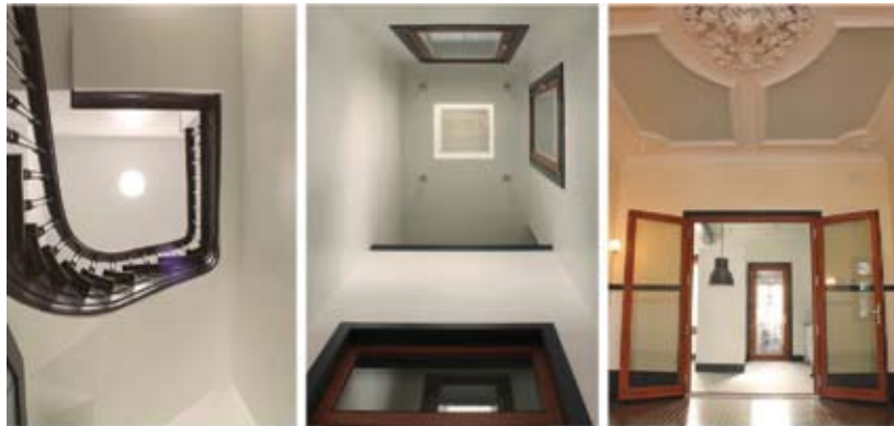
Left to right: Light wells bring natural light to center of building; Turret space utilized for passive cooling; Interior features such as plasterwork ceiling and staircase retained.
