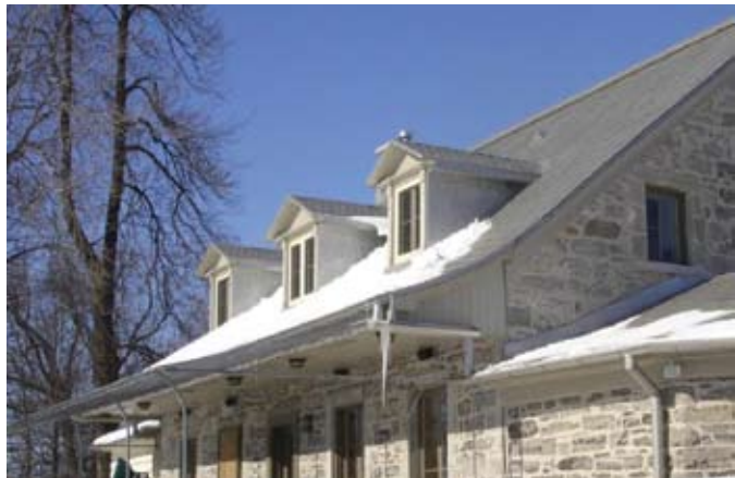
Deep projecting south-facing eave.
