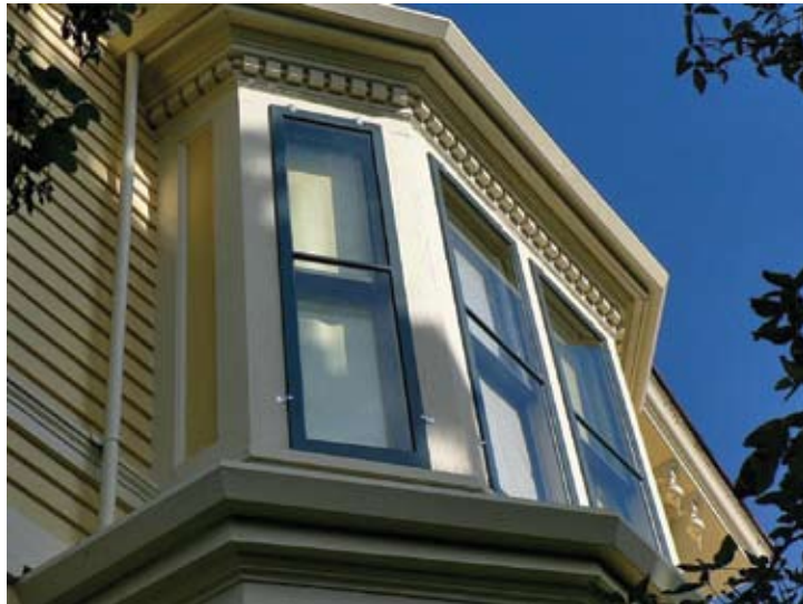
Figure 49 Rehabilitated exterior with windows. Windows feature exterior storm windows that can be removed depending on the season. Emily Carr House, Victoria, BC. Source: David Coulson Design
