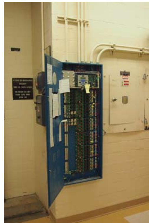
Figure 18 Light fixture management system. National Printing Bureau, Gatineau, Quebec. Source: M. Loiselle
