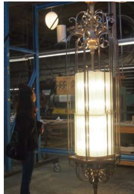
Figure 68 Rehabilitated chandelier with new wiring and energy efficient LED light sources. Sir John A Macdonald Building, Ottawa, ON. Source: MTBA Associates Inc.
