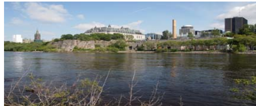
Figure 21 Cliff Street Heating Plant (on the right), district infrastructure for the Parliamentary Precinct, Ottawa, Ontario. Source: MTBA Associates Inc.
