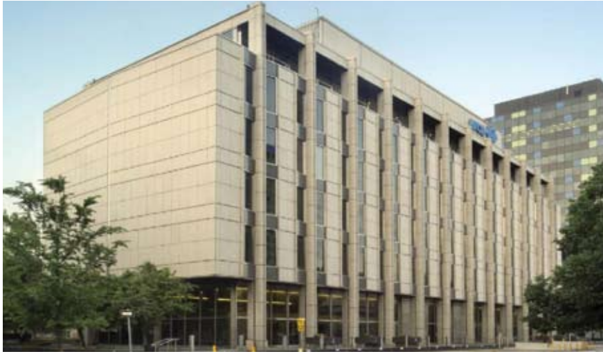
The Workers Compensation Board Building after retrofit. The stainless steel “expansion joints” are visible on the east façade and at the base of the columns.
