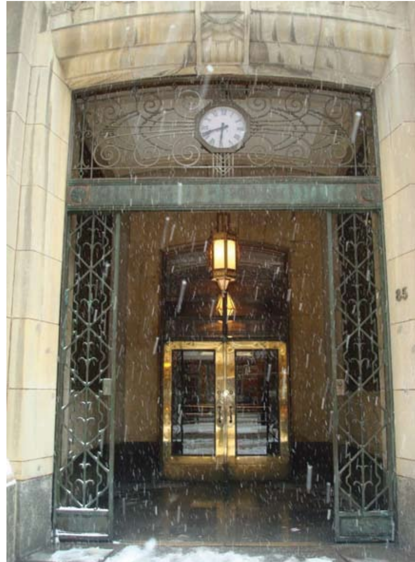
Figure 53 A portico and vestibule integrated into the entry sequence of a commercial building. The portico provides shelter from weather while the vestibule isolates interior from exterior. Aldred Building, Montreal, QC. Source: MTBA Associates Inc.
