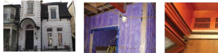
Left to right: The house prior to rehabilitation; Construction image showing insulation of interior wall assembly; Vent detail at south wall double window cavity.
