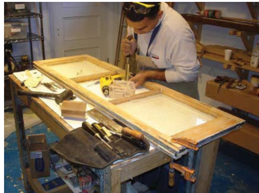
Figure 75 Wood window frame rehabilitation . Beaconsfield Yacht Club. Beaconsfield, QC. Source: FGMDA
