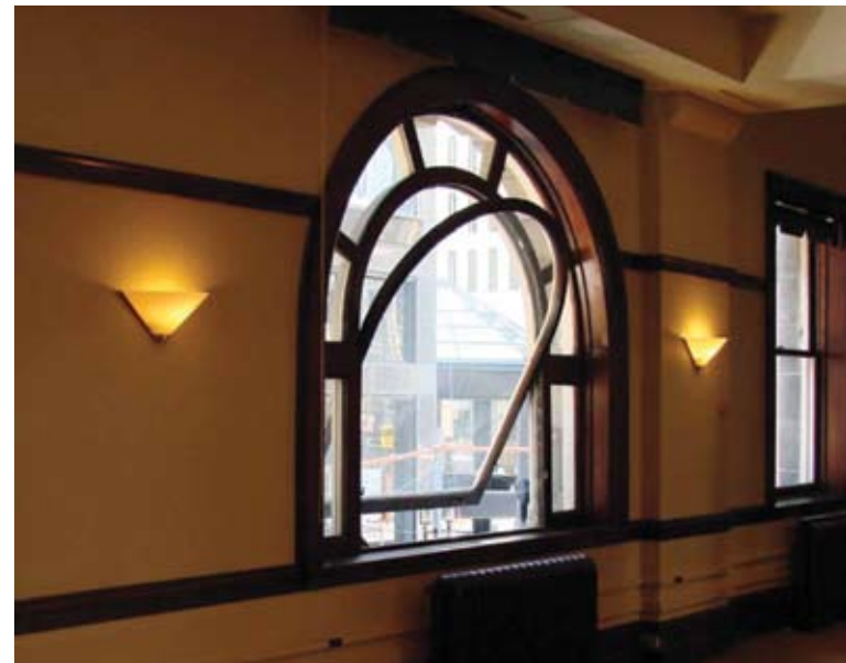
Figure 8 Operable windows in a heritage building that currently functions well for contemporary use and demands. (Ontario Heritage Trust, 10 Adelaide Street, Toronto)
