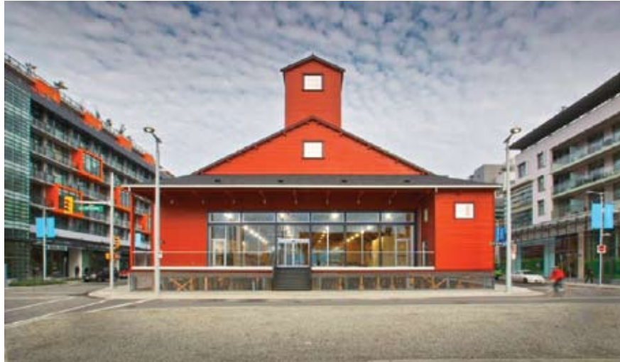
New large openings allow generous daylight into building
