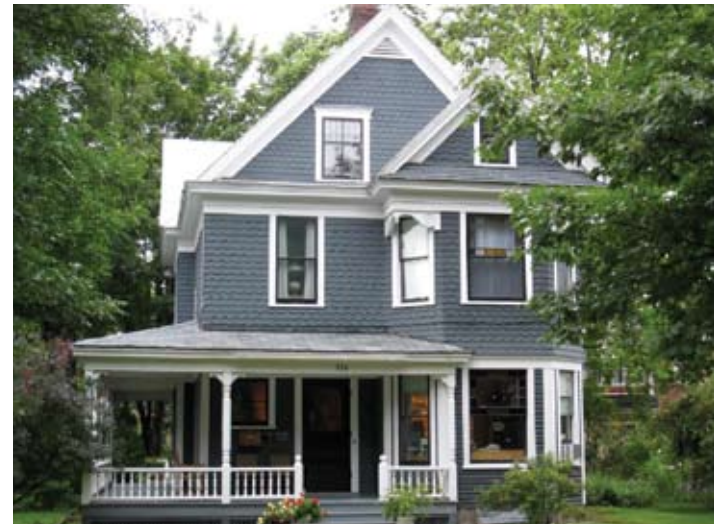
Figure 56 Front porches on early single-family residences such as this one in Fredericton, NB provide both shade and an opportunity for natural cross ventilation. Source: Shelley Bruce
