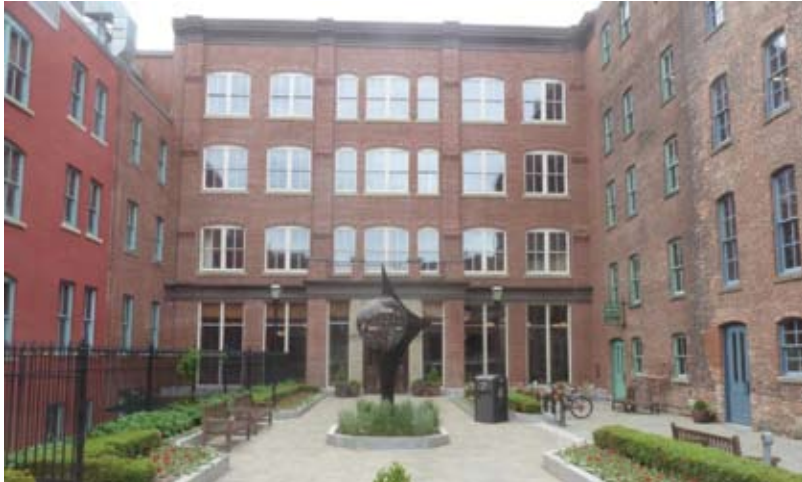
New south (rear) facade, designed sensitively with existing context, provides passive solar gain and a courtyard for outdoor activities. Source: Jim Bezanson
