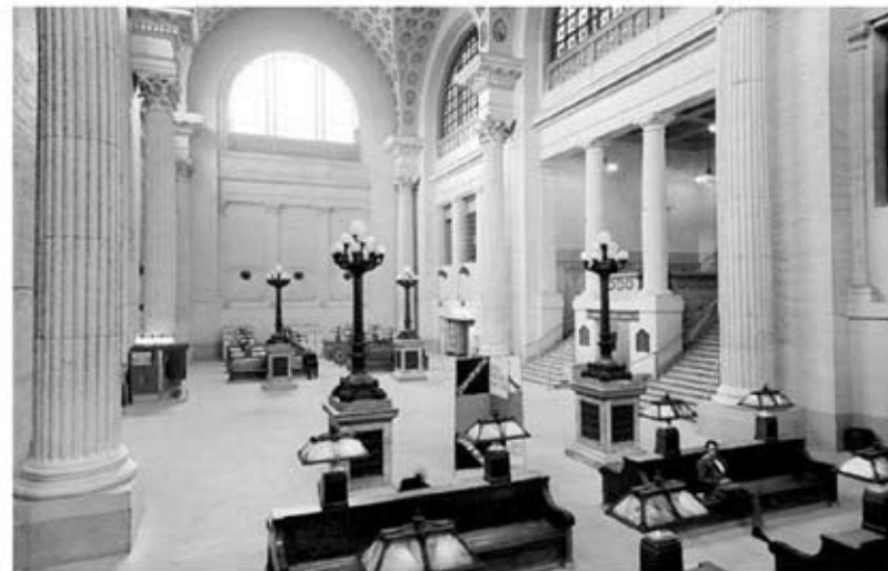
Figure 12 Waiting room of the 1912 Union Station, Ottawa. Image c.1950, showing HVAC systems integrated to furniture and design elements (i.e. benches and lighting pedestals) Source: Archive, National Capital Commission
