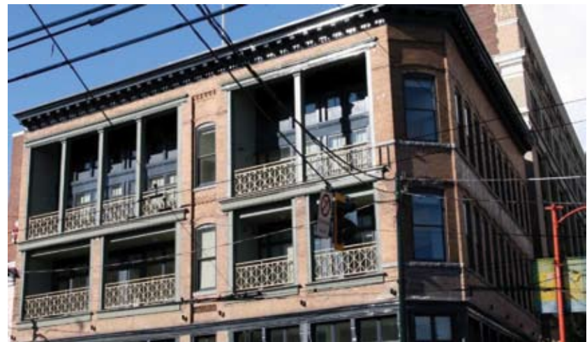
Figure 55 Recessed balconies on a street-facing elevation were retained during the overall rehabilitation of this building. Chinese Freemasons Building, Vancouver, BC. Source: Shelley Bruce
