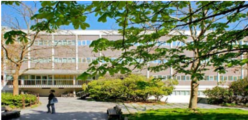
Figure 25 Rehabilitated exterior assembly. Friedman Building, University of British Columbia Source: Acton Ostry
