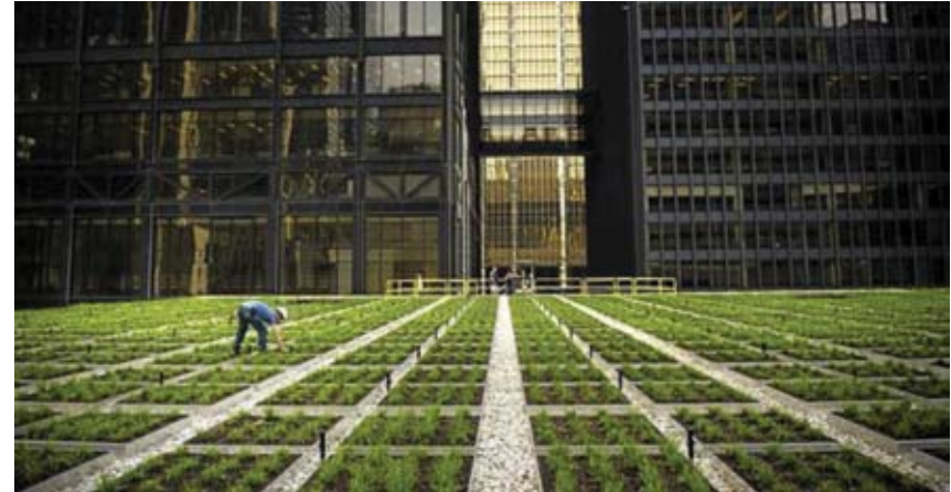
Figure 41 New Banking Pavilion green roof. The grid used for the green roof mirrors the lighting layout of the pavilion's ceiling below, harmonizing with character-defining design attributes. The green roof reduces heat island effect, provides insulation, reduces and/or slows water run-off, while having no negative impact on heritage value. This upgrade was completed as part of a comprehensive multi-building rehabilitation and upgrade to this icon of Modern architecture in Canada. Toronto Dominion Centre, Toronto, Ontario. Source: Globe and Mail
