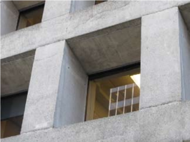
Figure 80 Poured-in-place exterior concrete facade. MacMillan Bloedel Building
