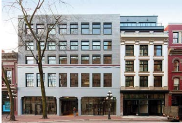
Figure 48 Rehabilitated storefronts with transoms. The taller storefront glazing provides light deeper into the ground floor storefronts. Vancouver, BC. Source: Acton Ostry.
