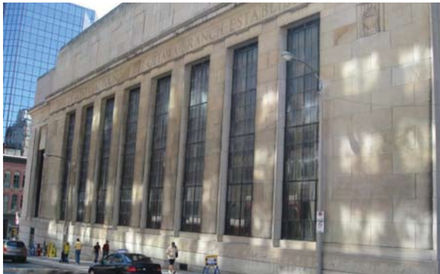
Figure 47 These large bronze-framed double-layered windows (storm and primary) were retained and rehabilitated, maintaining the primary source of light as when the building was constructed. Energy upgrades were limited to new gaskets on the interior operable windows which increased the lifespan of the windows Sir John A Macdonald Building, Ottawa, ON. Source: MTBA Associates Inc.
