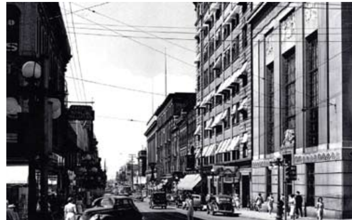
Figure 50 Historical photograph of the Booth Building (second building from the right) on Sparks Street in Ottawa. It is important to recognize windows were historically composed of a number of parts that contributed to their performance. In this case, the south facing windows were protected from increased heat gain by fabric awnings, accessible through operable windows. Booth Building, Ottawa, ON. Source: Ottawa AA
