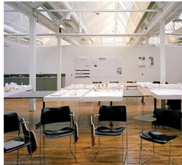
Figure 69 Hardwood flooring and ceiling cladding were retained as part of rehabilitating a former riverside factory into an institutional building. Note the effective use of natural light with clerestory windows, which helps reduce energy costs. University of Waterloo School of Architecture, Cambridge, ON. Source: Doors Open Ontario
