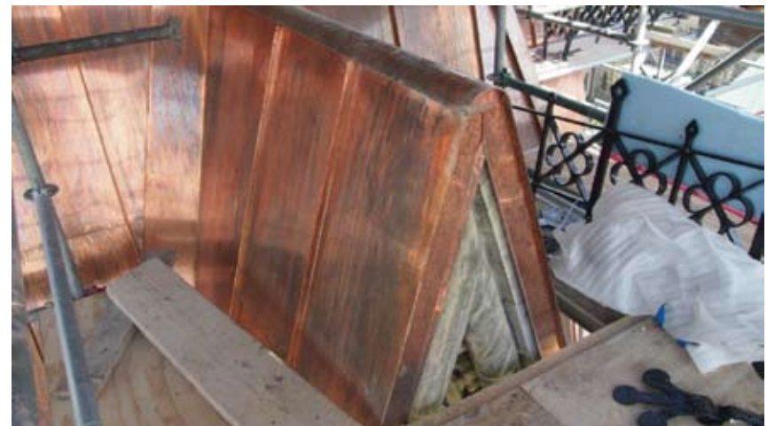
Figure 40 Modified fascia height to accommodate new insulation. Modifications achieve building envelope performance improvements with very limited visual impact. East Block, Parliament Hill, Ottawa, ON. Source: MTBA Associates Inc.
