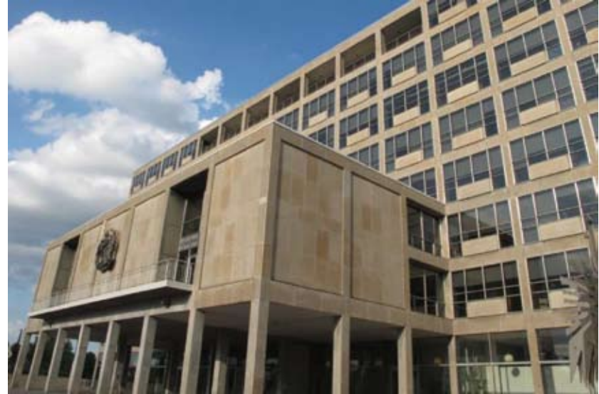
Figure 54 The projecting Council Chamber, complete with balcony, shelters the main entry below. Former Ottawa City Hall, Ottawa, ON. Source: MTBA Associates Inc.
