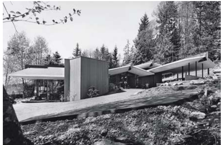
Figure 36 Deep, low slung roofs over both interior and exterior space provide both shading and the home's distinctive form. Forest House, Ron Thom. Source: AZN Modern
